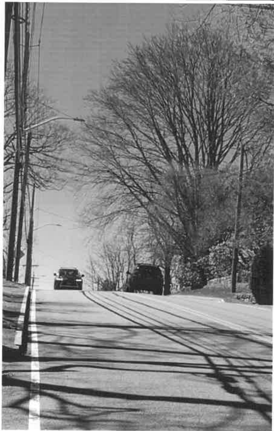
Example of poor sight distance along Ridgeway
